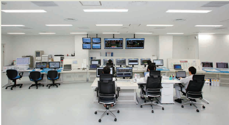
Central Control Room
