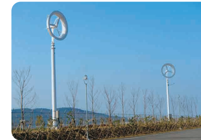
Generating capacity : 2 units, 5 kW each
